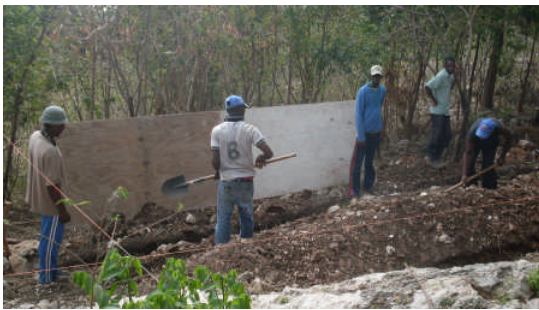
Men working on bathroom
