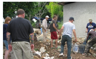
The foundation being laid for a new bathroom.
