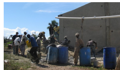
Mixing the cement by hand and then moving via bucket line
